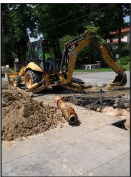
Phase 1 of this project included the upgrade of the water main running underneath Steamboat Road. The new 8-inch water main was installed by the Great Neck Water Authority, and was completed in August of 2012.
